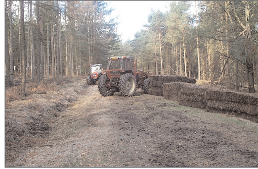
Contractors stockpiling heather bales along ride edge ready for mire restoration and drain infill works
