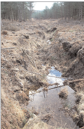
Over deepened ditch cleared ready for infill works.
