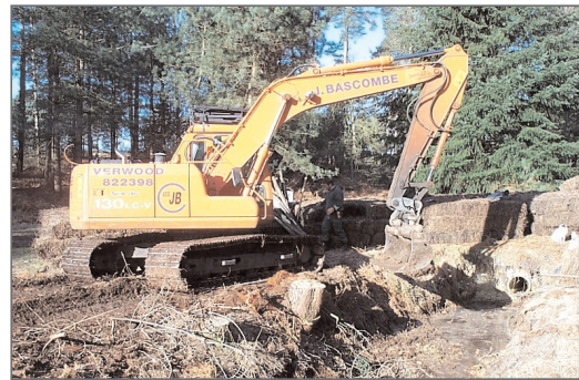
Contractors infilling drainage channel with heather bales
