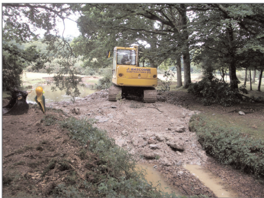
Constructing clay plug - Markway
