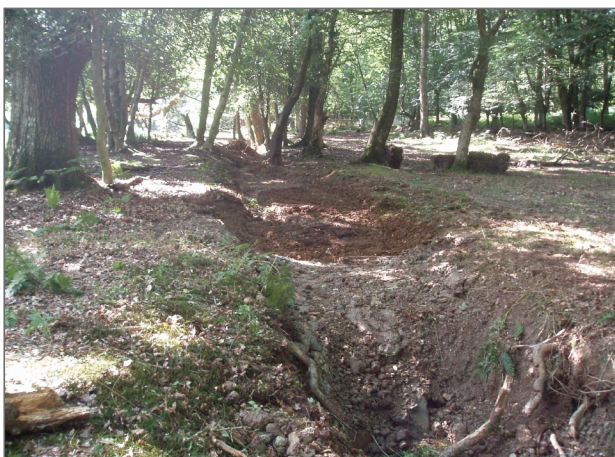
Installing clay plugs
