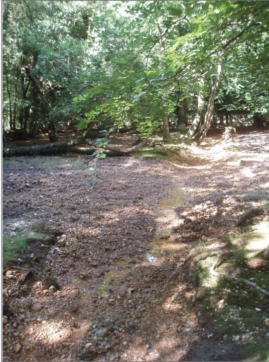
Ditch post restoration
