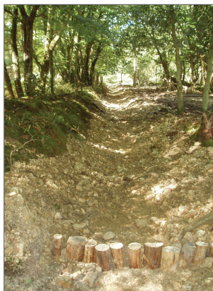
Chestnut post dams to prevent movement of material
