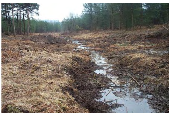
Over deepened ditch cleared ready for infill works.
