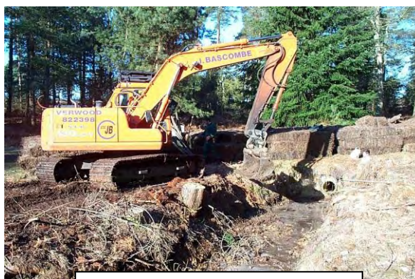
Contractors infilling drainage channel with heather bales
