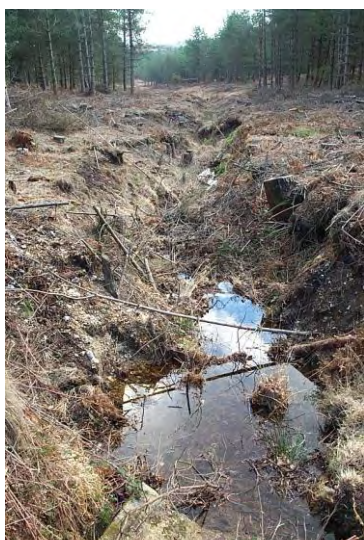
Over deepened ditch cleared ready for infill works.
