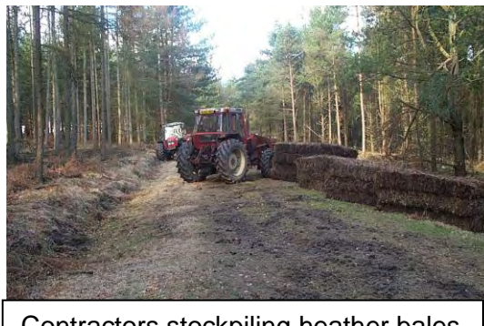
Contractors stockpiling heather bales along ride edge ready for mire restoration and drain infill works
