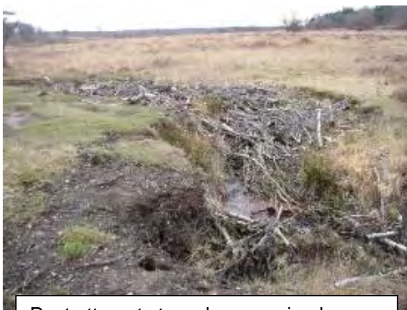
Past attempts to reduce erosion by infilling with branchwood failed
