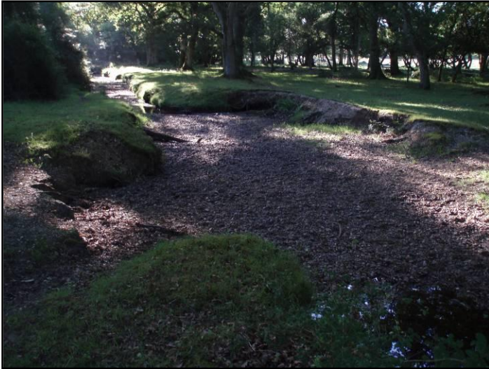
Photo 1 – Markway, July 2006 Artificial straightened drain which was limiting floodplain inundation and with the erosive force constricted to the channel. Significant deposition of upstream material is shown here.
