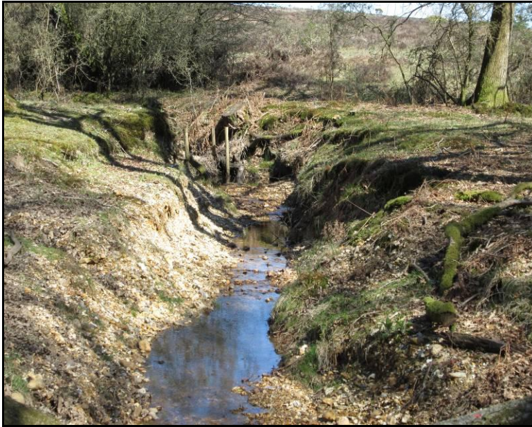
Photo 1 – Buckherd Bottom, March 2013 Eroded channel through pasture woodland, before restoration.
