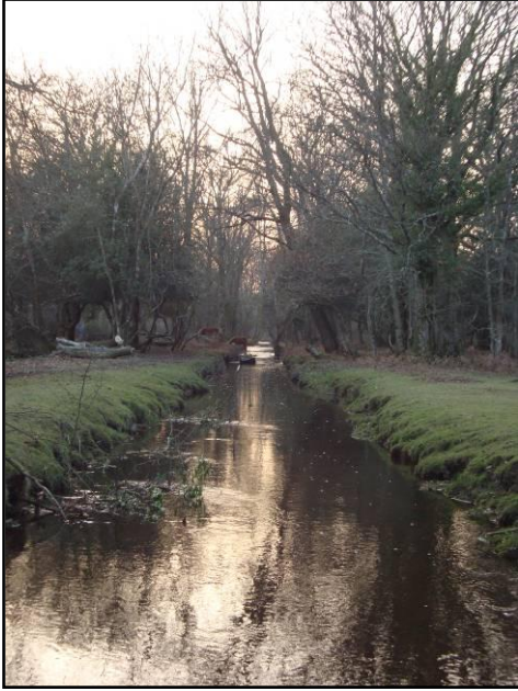
Photo 1 - Fletchers Thorns, February 2011 Artificial straight, wide drain which was limiting floodplain inundation, with the erosive force constricted to the channel.
