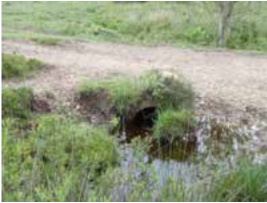
Latchmore - 1.3 - 13 - upstream (culvert and footpath) - 20130621
