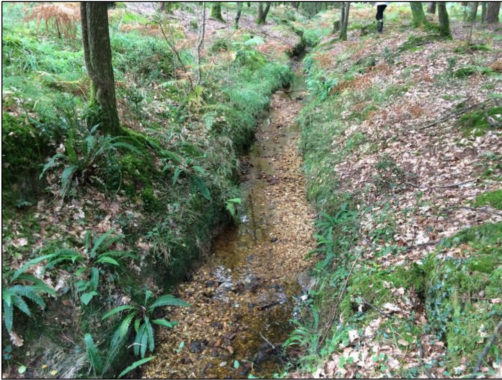
Figure A14.3. Habitat immediately downstream of culvert at South Oakley 1.
