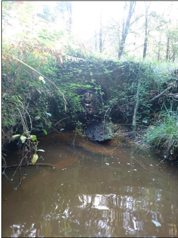
Figure A14.2. Downstream end of culvert at South Oakley 1.
