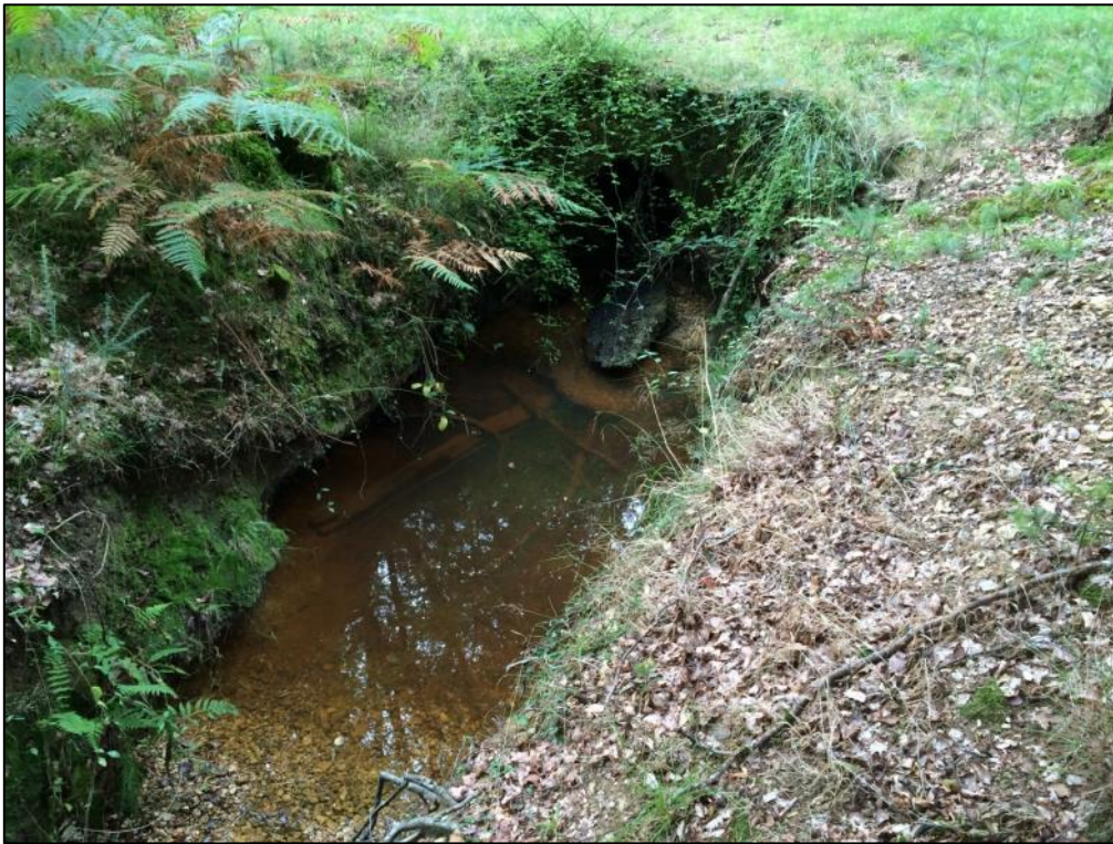
Figure A14.1. Downstream end of culvert at South Oakley 1.
