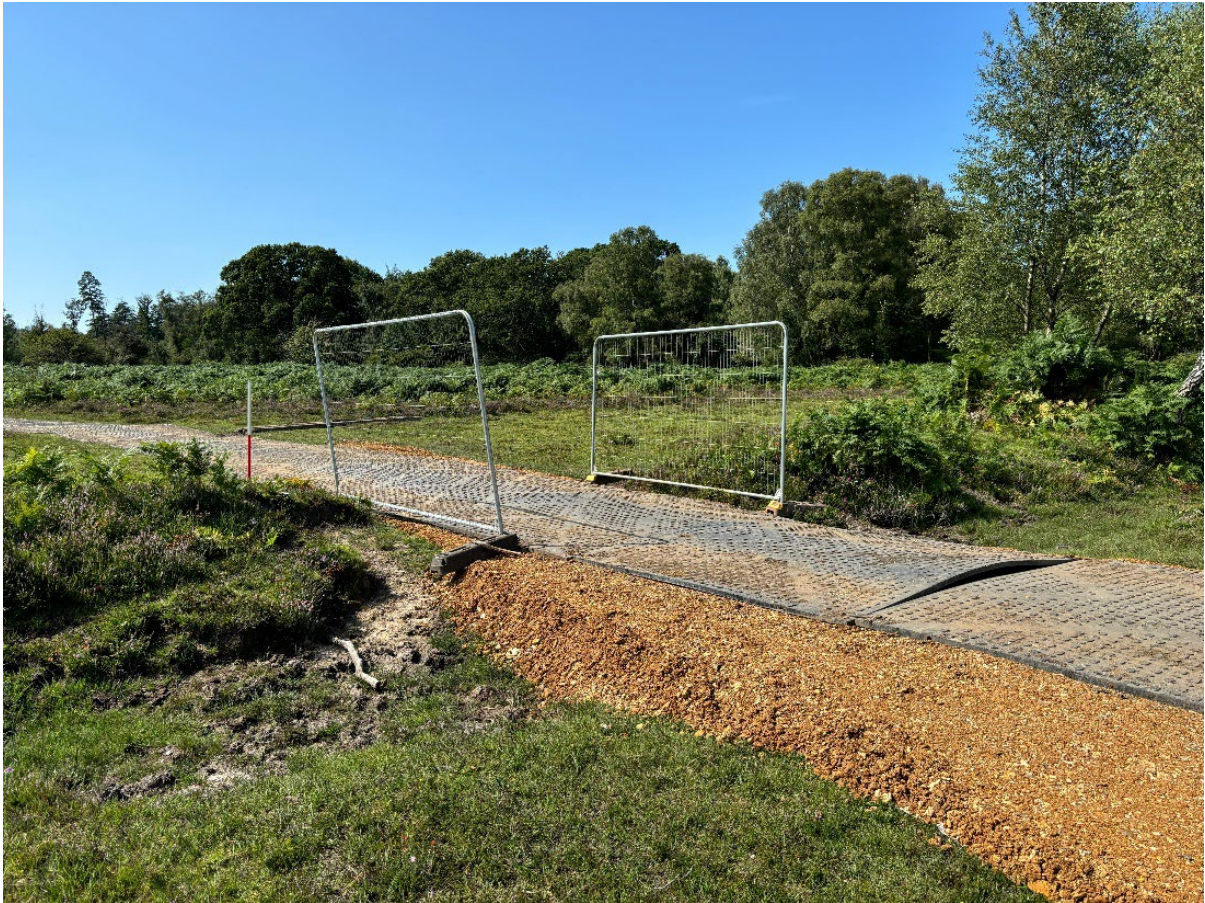
Figure 3: Completed engineered surface to protect the Scheduled Monument, with temporary road matting on top.
