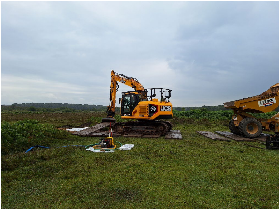
Figure 2: Engineered surface being laid to protect the Scheduled Monument from further damage.
